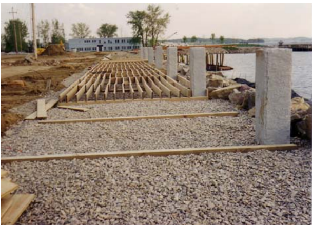
View of Boardwalk Framing
