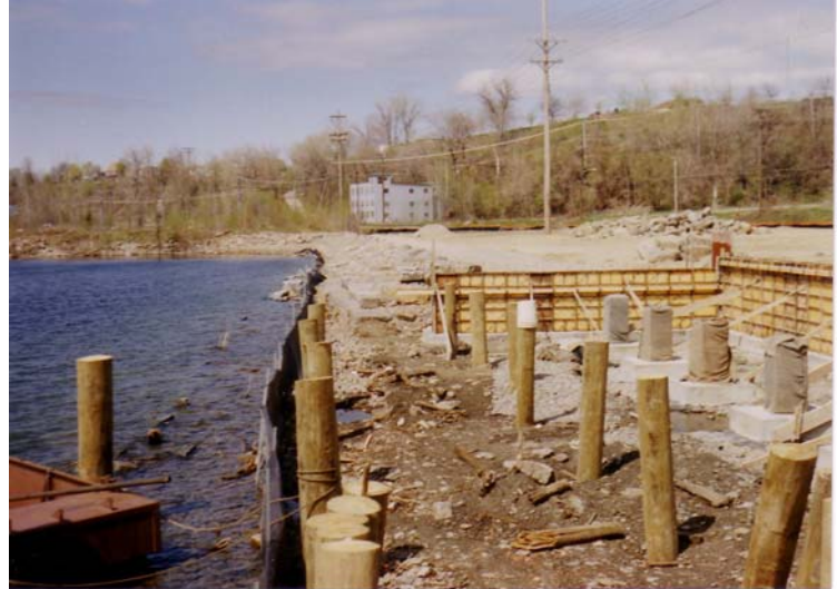
View of Timber Piles for Promenade
