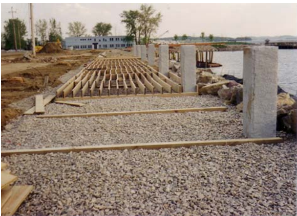
View of Boardwalk Framing
