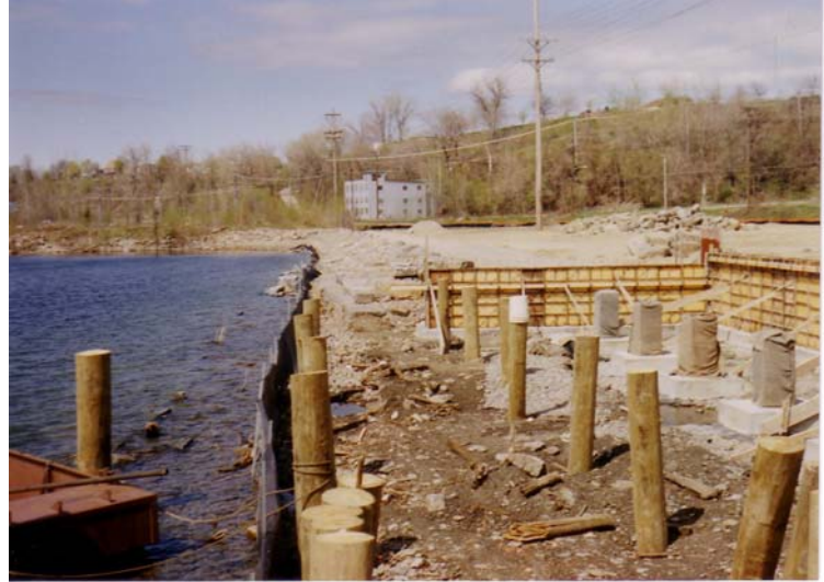
View of Timber Piles for Promenade
