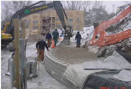
MSE Wall at Parking Lot (Southeast)
