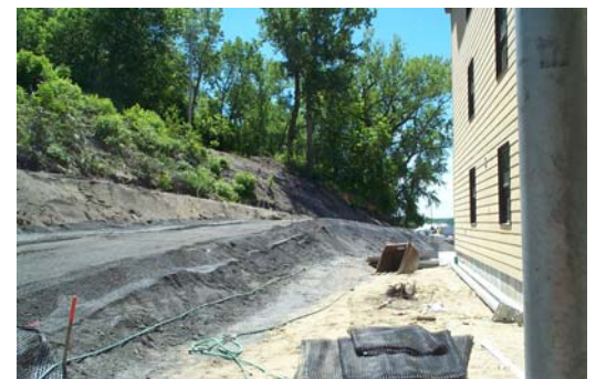
Reinforced Slope (East)
