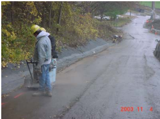
New Depot Street Paved Swale
